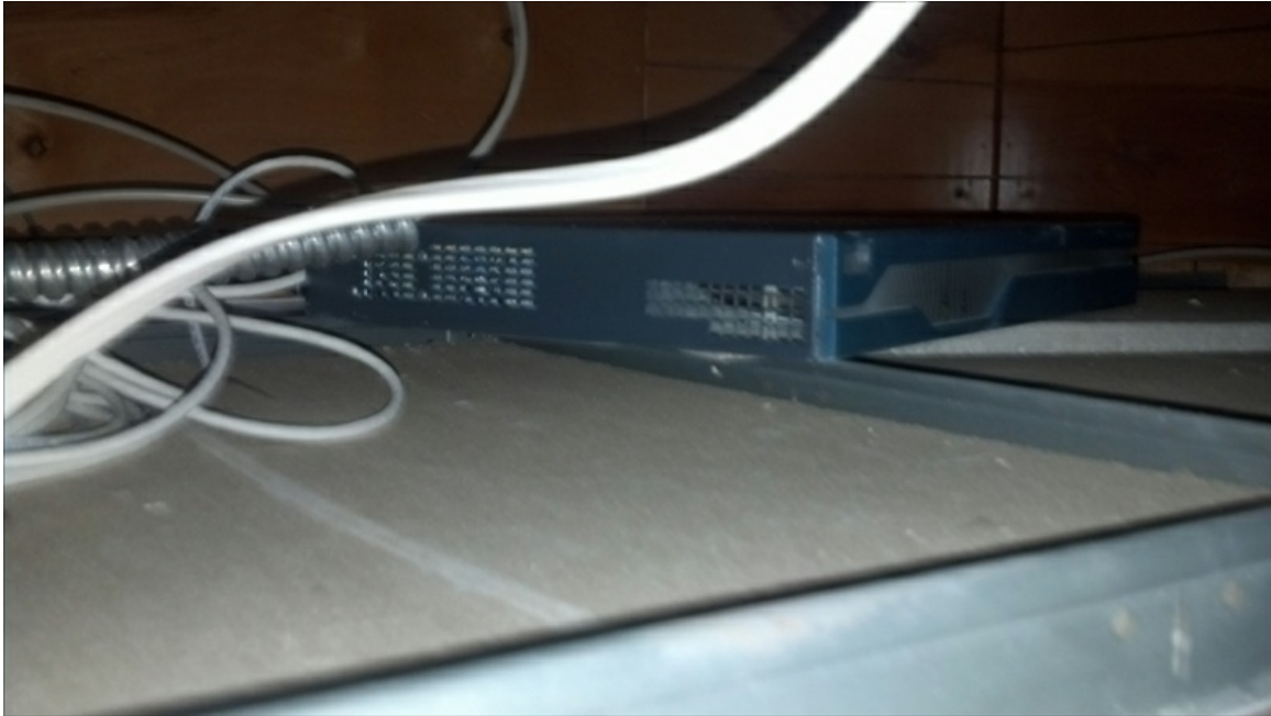
Figure 2-15 Incorrect Router Placement
